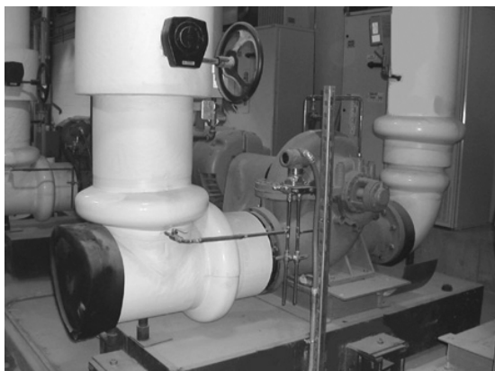
Fig. 4 LS pump in a commercial building application
