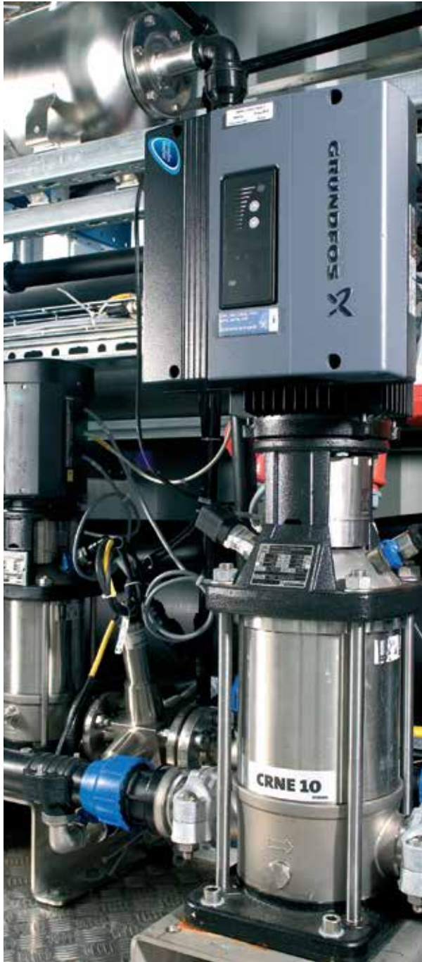
CRE pumps represent the union between high quality pumps and superior variable-speed motors. This plays a vital role in process control, surveillance and protection.
